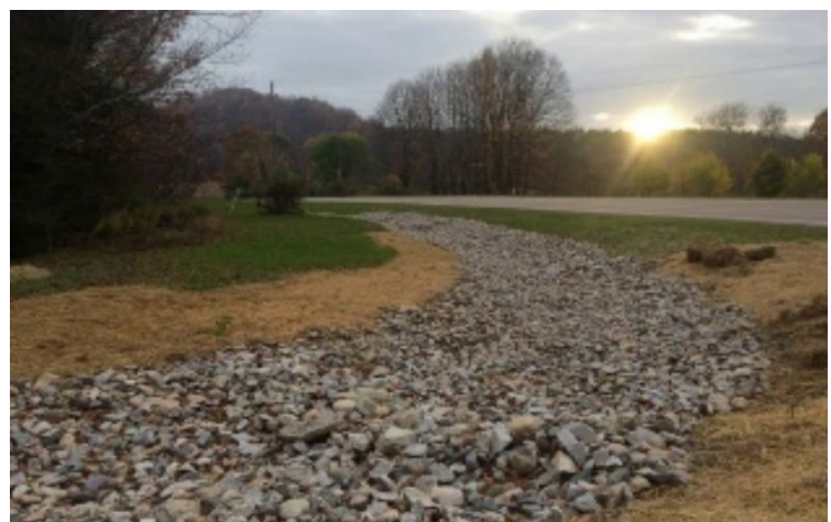
Figure 21. (Left) Stormwater runoff from agricultural fields and private land caused significant gully erosion into the West Branch of the New Haven River in the town of Bristol. (Right) The gully was restored and stabilized with a stone lined swale with check dams and plantings in March 2020. Implemented in partnership with Otter Creek Natural Resources Conservation District and funded by the Clean Water Initiative Program.
