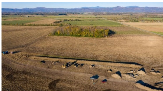
Figure 22. A wastewater disposal mound is a soil absorption system placed above the natural surface of the ground. The Town of Addison installed a community wastewater disposal mound system to treat municipal waste in June 2019. The project was financed by the Clean Water State Revolving fund.
