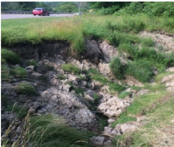
Figure 21. (Left) Stormwater runoff from agricultural fields and private land caused significant gully erosion into the West Branch of the New Haven River in the town of Bristol. (Right) The gully was restored and stabilized with a stone lined swale with check dams and plantings in March 2020. Implemented in partnership with Otter Creek Natural Resources Conservation District and funded by the Clean Water Initiative Program.
